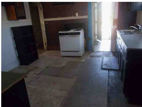
Kitchen - Front Unit
