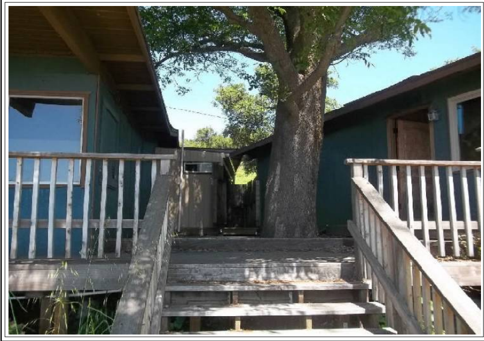
FRONT DECK, ENTRY TO HOUSE AND SHOP
