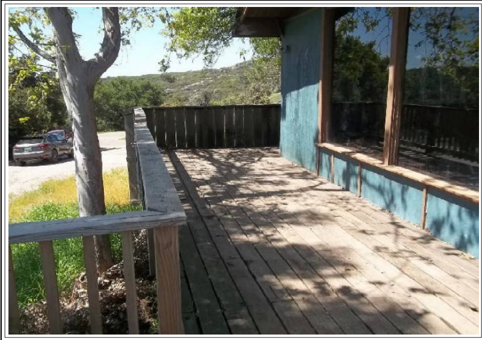
FRONT DECK OF HOUSE
